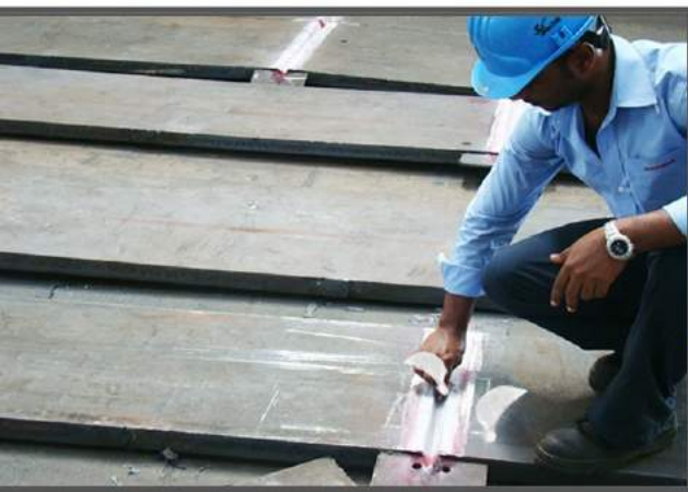
Liquid Penetrant Test
